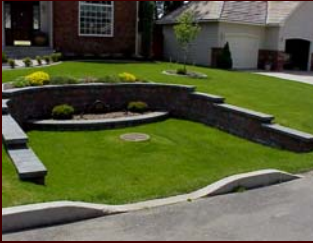
An example of a swale with a drywell.
